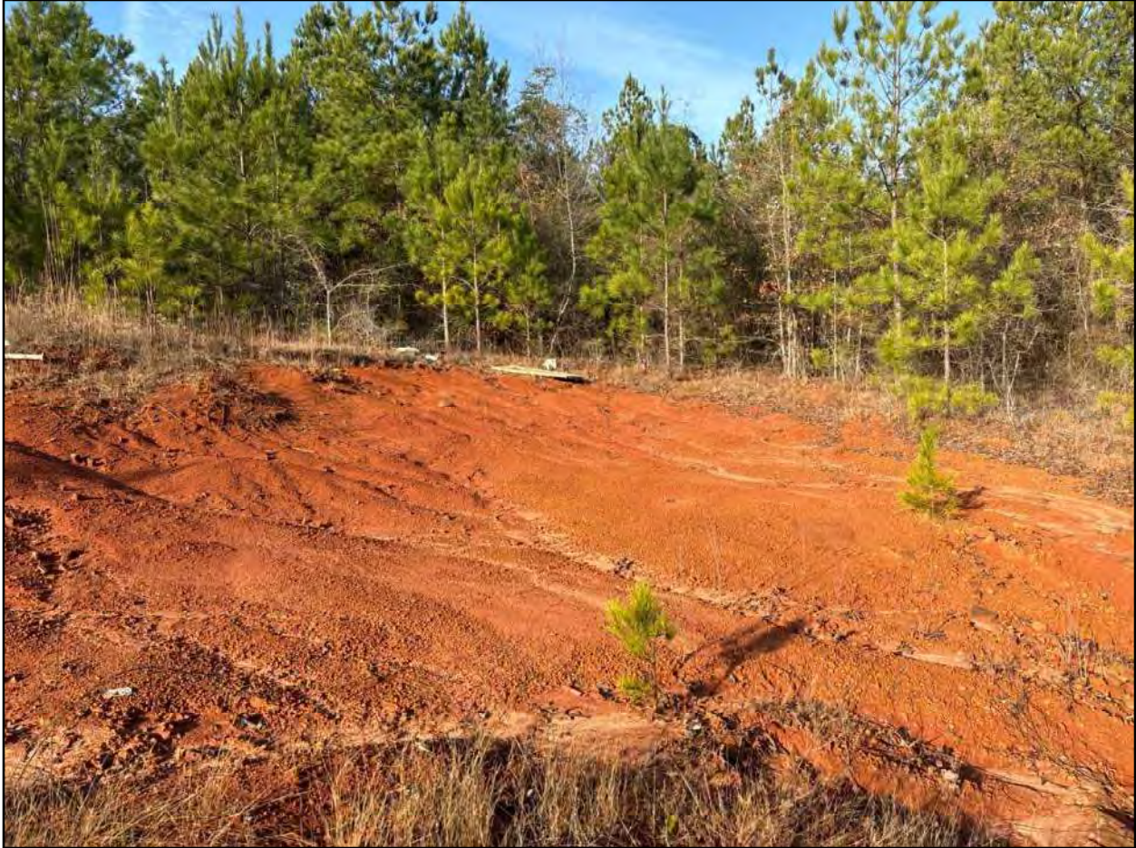
Figure 3.1 Erosional surface near a road through tree-covered terrain in Parcel 68 1 of the Heart Pine Solar project area.
