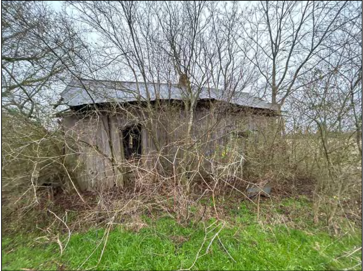
Figure 3.7 Abandoned wood plank farmhouse with brick chimney and loft at Locus 4 in the Claudine Morgan parcel of the Heart Pine Solar project area.
