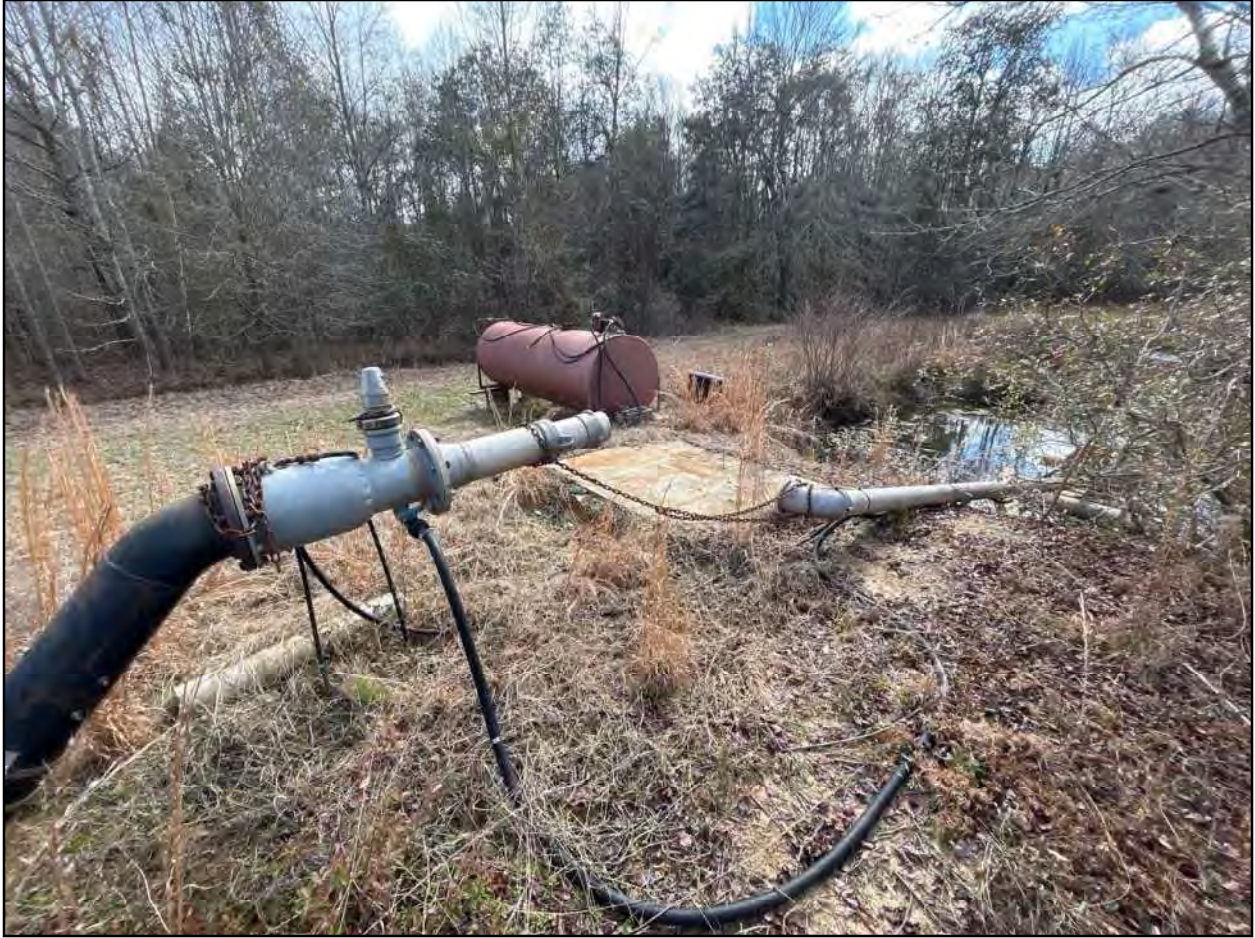
Figure 3.2 Pipes and a storage tank near Heritage Ford Creek in the Claudine Morgan parcel of the Heart Pine Solar project area.
